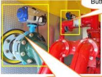
Water Outlet Control Valve: Button 1 ON: Valve open Button 1 OFF: Valve close
